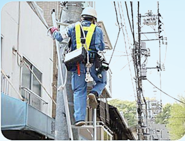
Optical fiber emergency repair
