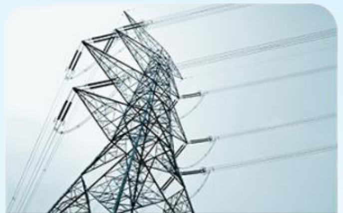
Optical fiber wiring
